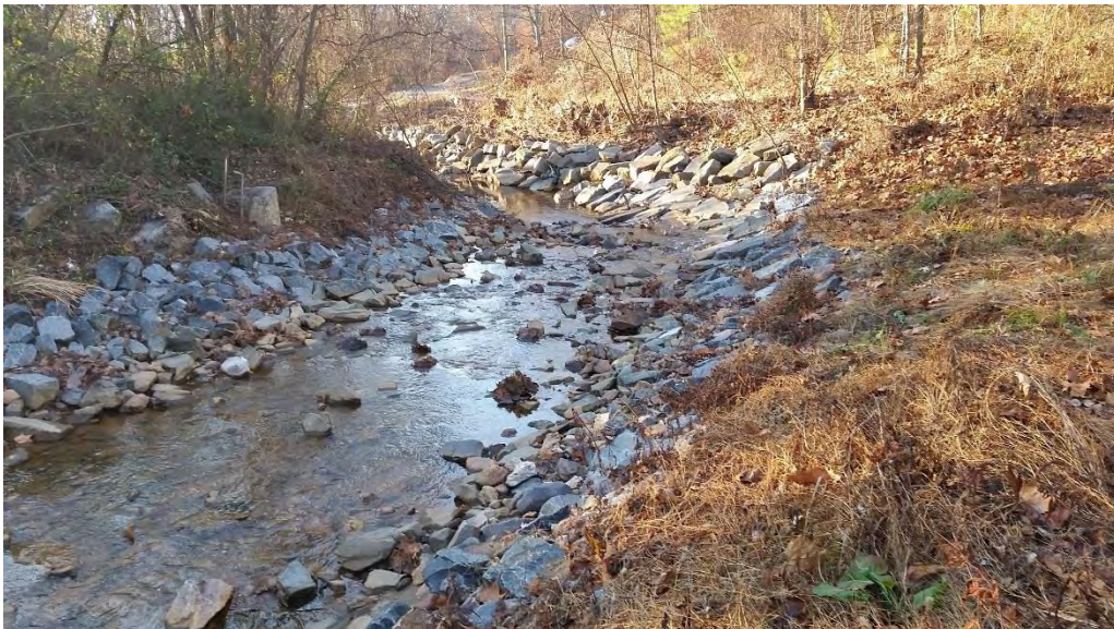
Figure 15: Looking downstream from most recent bed and bank armoring. Sampling reach lies downstream from where photo location.
