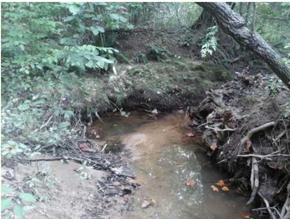
Eroded area of stream channel
