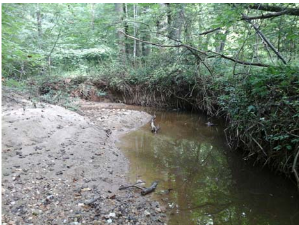
Impacted stream reach showing undercut bank
