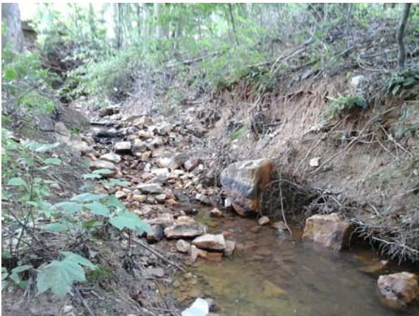
Exposed and eroded bank
