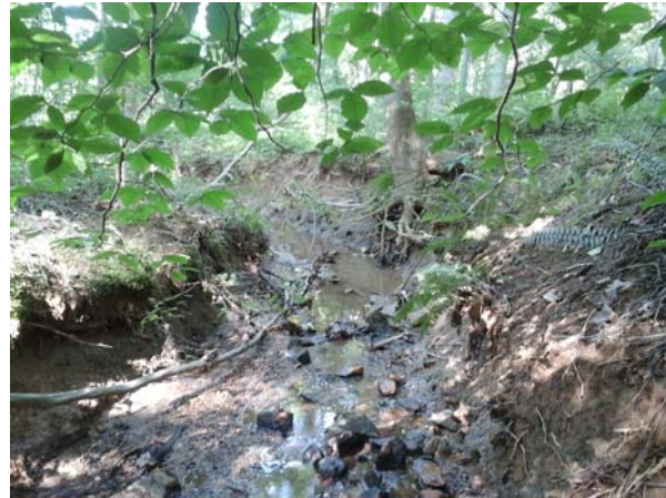
Unstable section of reach showing active erosion
