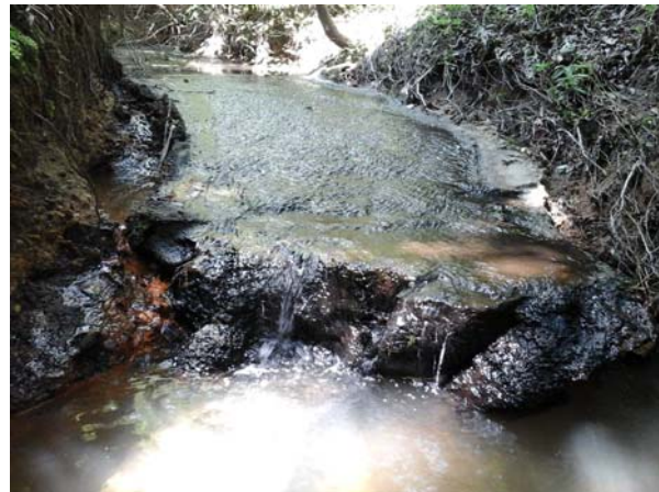
Restoration opportunity showing concrete stream bottom
