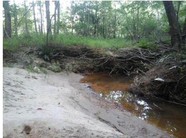
Eroded outer bank of stream channel, exposing root systems
