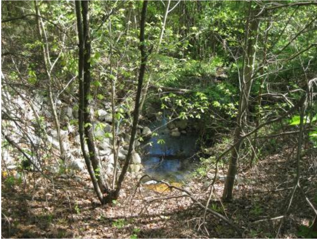
37. Facility 163. Looking at stable receiving channel immediately downstream of facility.
