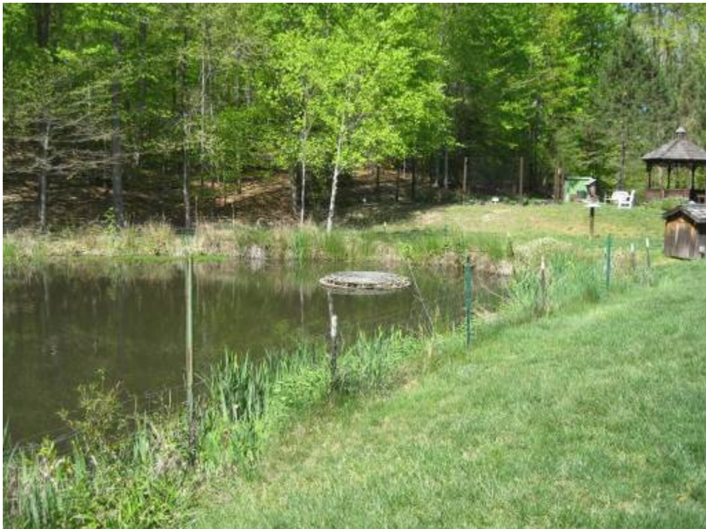
24. Facility 5255. Looking at riser and perimeter fence.
