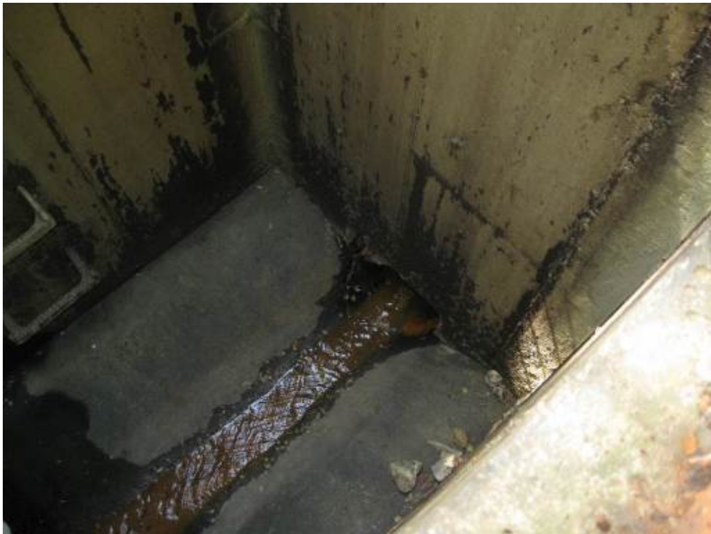
18. Facility 481. Looking in riser at low flow orifice.
