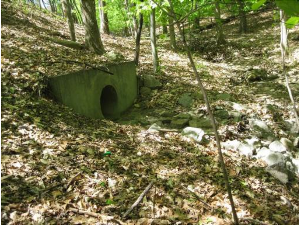
23. Facility 5147. Looking immediately downstream of facility outlet as it drains into receiving channel which is stable.
