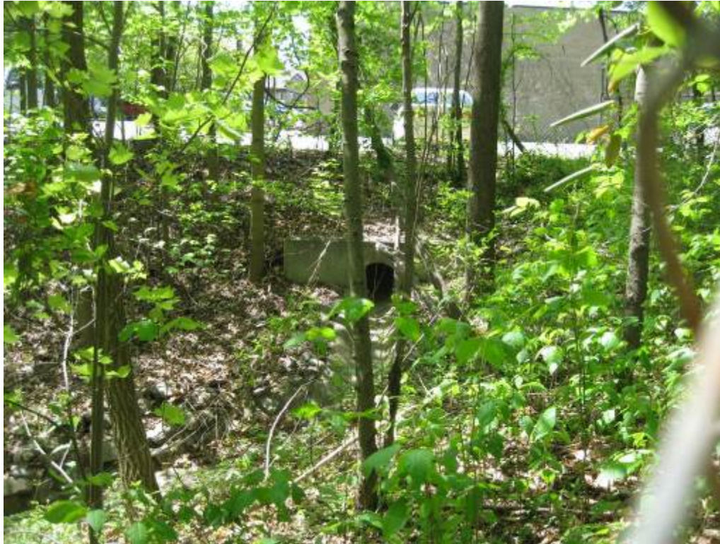
21. Facility 5147. Looking at pipe that drains parking lot runoff into facility.
