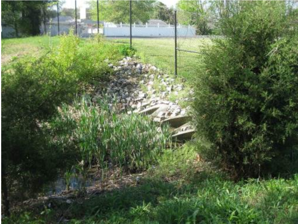
63. Facility 5153. Looking at stable inlet from school buildings.
