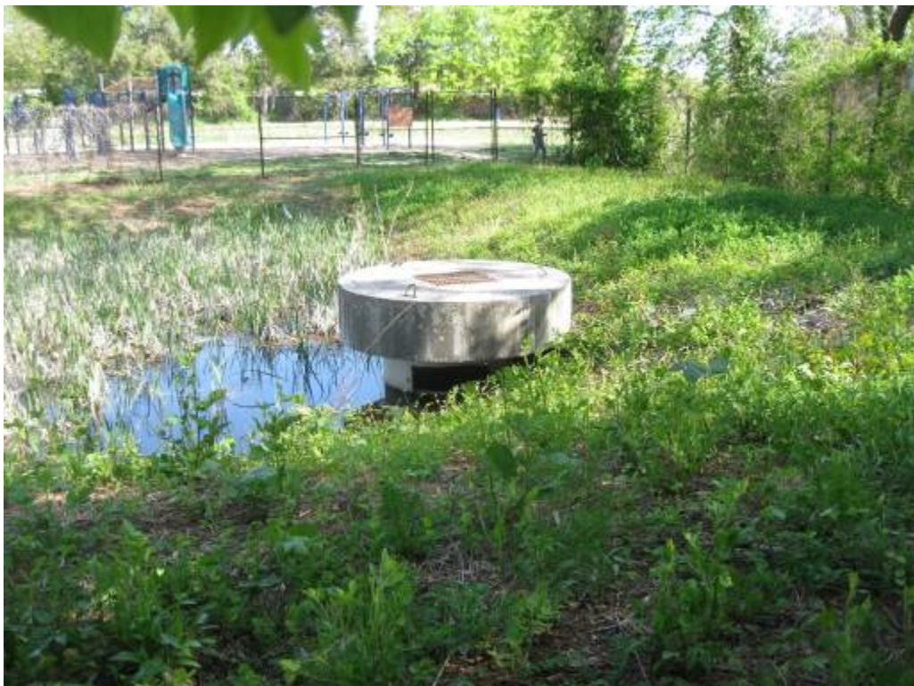
62. Facility 5153. Looking at concrete riser. Facility treats school lot, including buildings, parking lot, playground, and turf grass.
