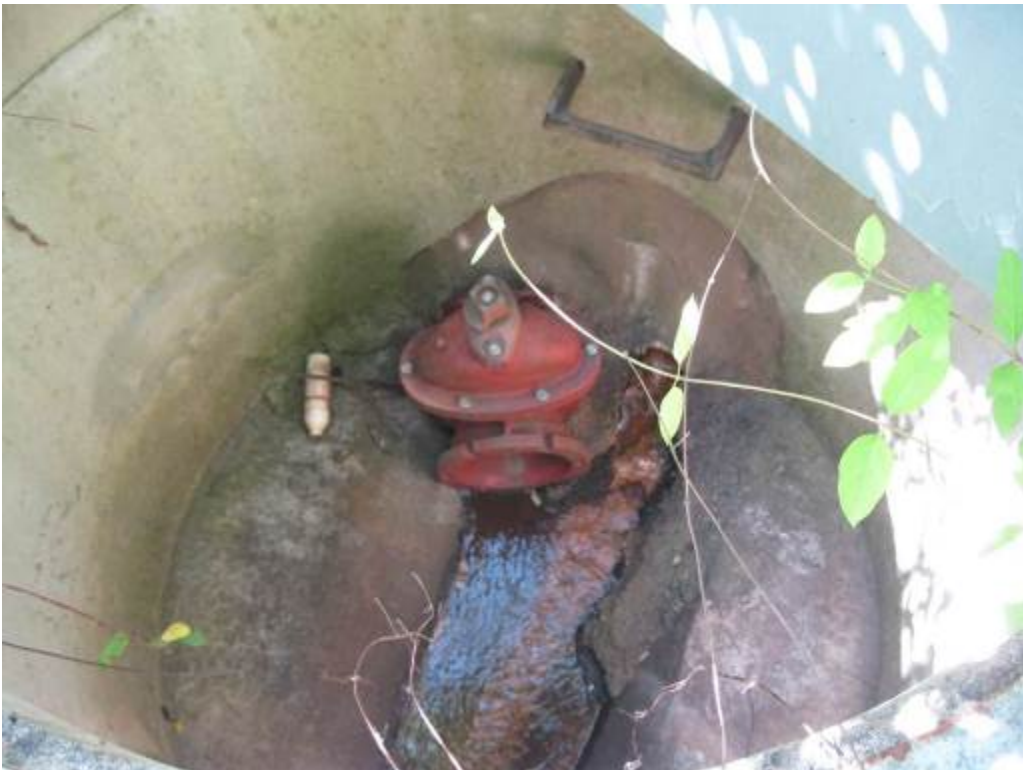
34. Facility 163. Looking in riser at maintenance valve and low flow orifice.
