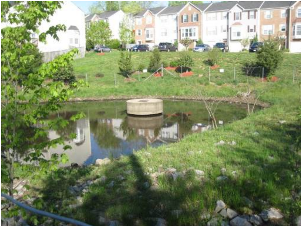
46. Facility 454. Looking at riser structure from the emergency spillway.
