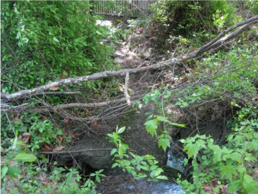
65. Facility 5153. Emergency spillway drains to existing asphalt channel.
