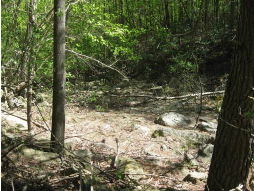
15. Facility 28. Looking at grouted natural boulder in emergency spillway.
