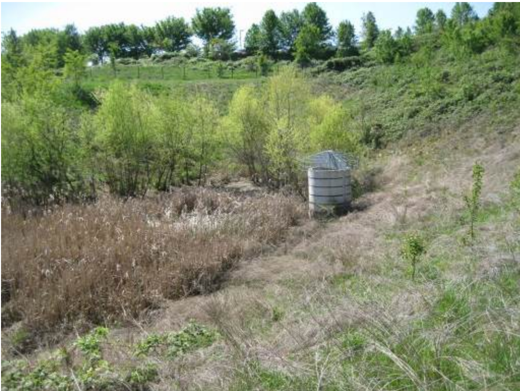
66. Facility. 5400. Looking at riser and wet ponding area.
