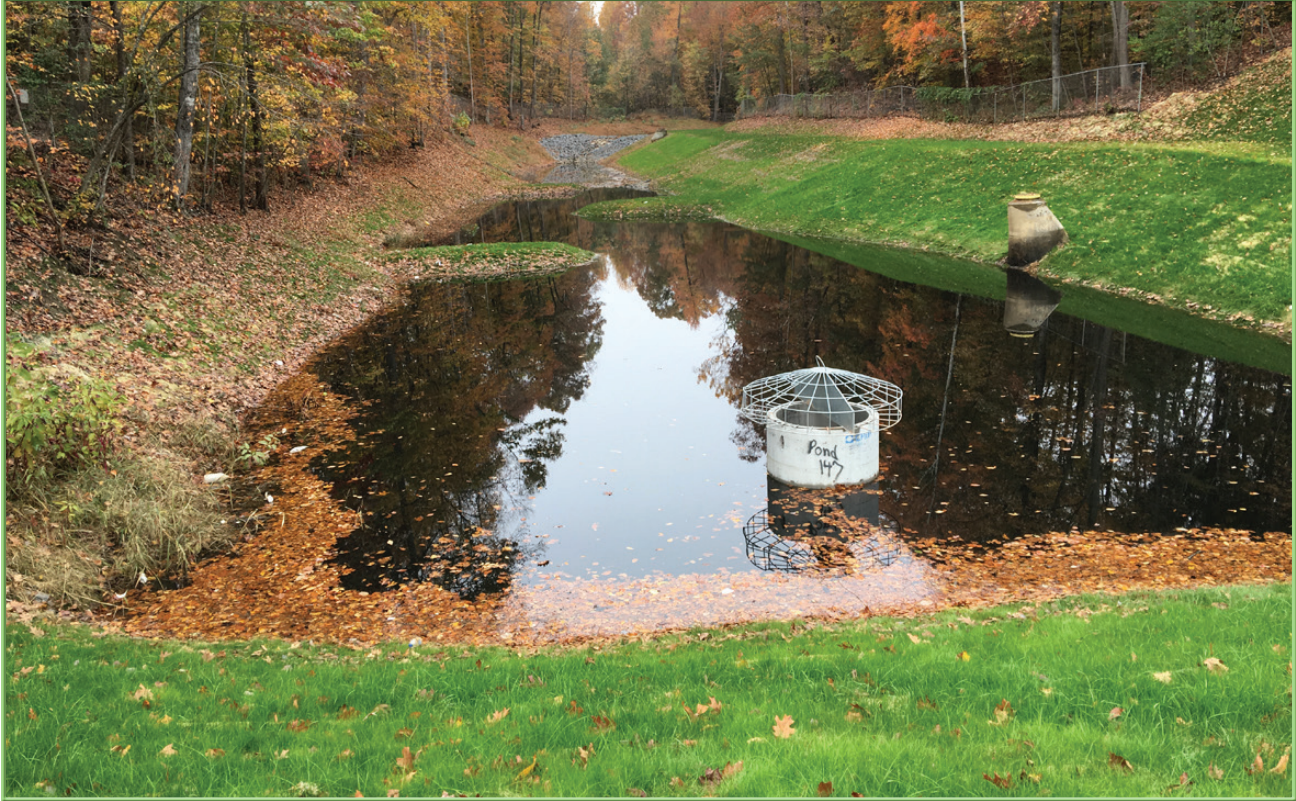
Powells Creek Watershed Water Quality Retrofit
