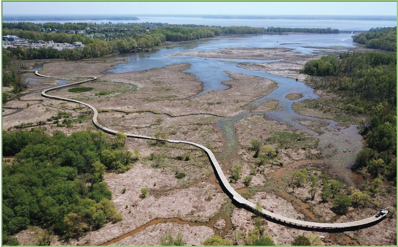
Potomac Heritage National Scenic Trail - Neabsco Creek Crossing
