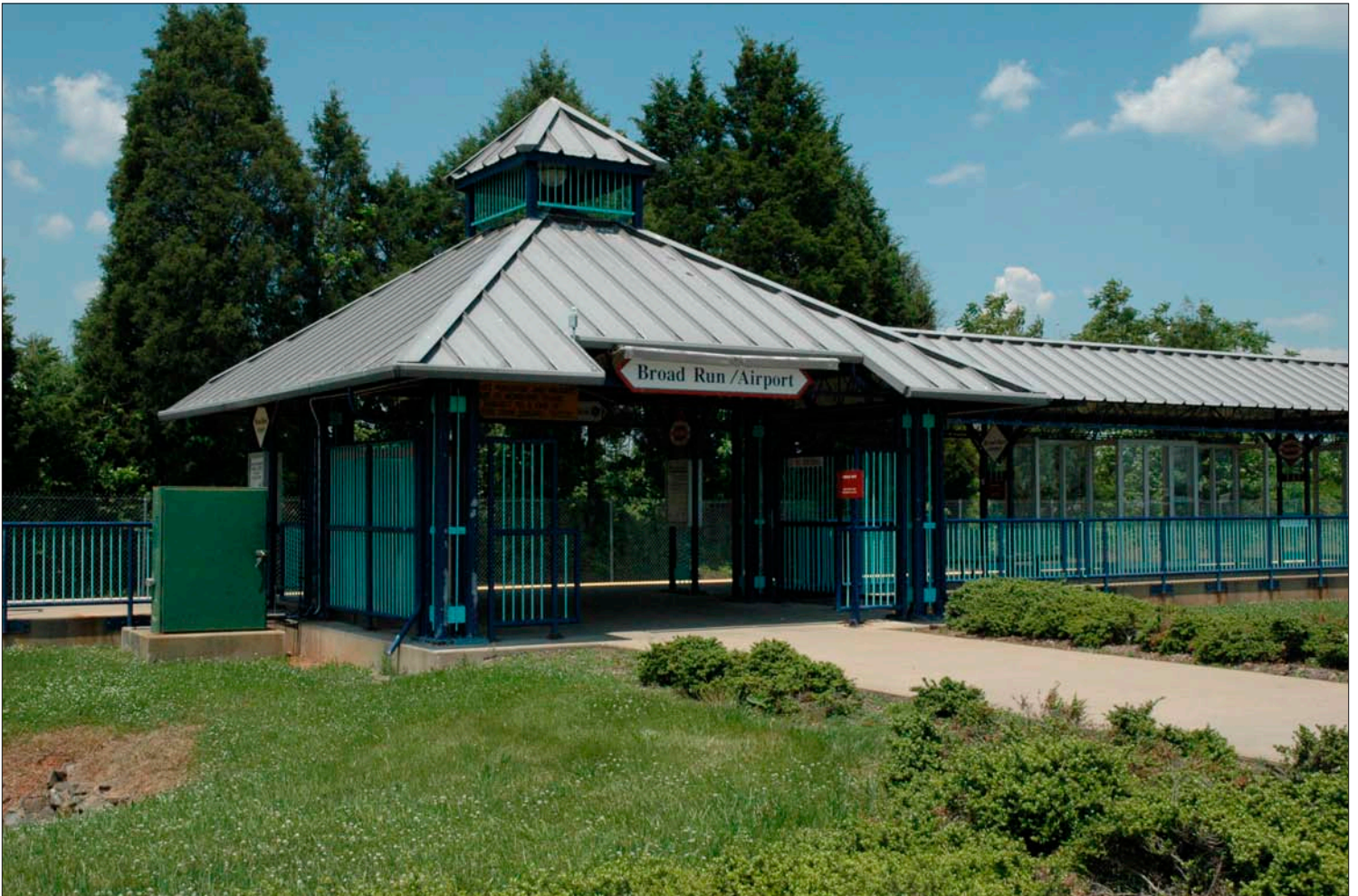
Broad Run Commuter Rail/VRE Station
